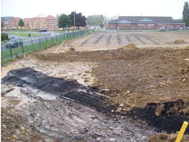
Outcrop of coal close to the surface which would be sterilised without prior extraction and has the potential to cause instability for surface development
